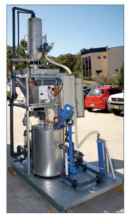
Fluoride solution can be gravity fed or transferred to the injection point via a ProMinent Spectra® progressive cavity pump with controlled flow.
